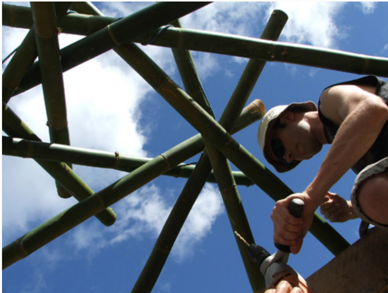
Building on site with lightweight bamboo roof structure.
